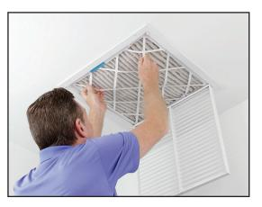
While they look impervious, air can move through under pressure leaving its airborne cargo trapped. Pleated filters are probably better.
